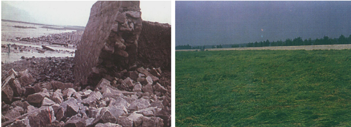
Fig. 2 – The sea dike without S. alterniflora vegetation in front was crushed (left) and the sea dike with S. alterniflora vegetation in front was saved (right) in Dongtang district of Wenzhou City, China when the 17th strong typhoon attacked the whole seashore in 1994. Photographs: L. Min.
